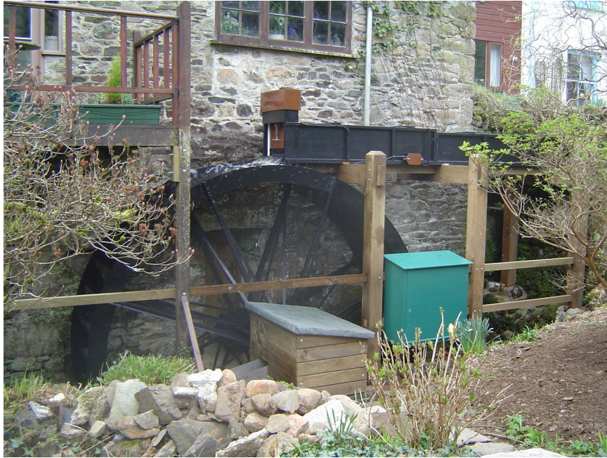
Lydia Mill: 3.86m diameter steel wheel, 70 litres/s, 1.8kW, up to 10,000kWh per year.
